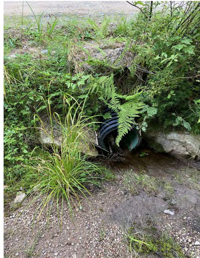
Photo 1: Culvert at the crossing, no water.
