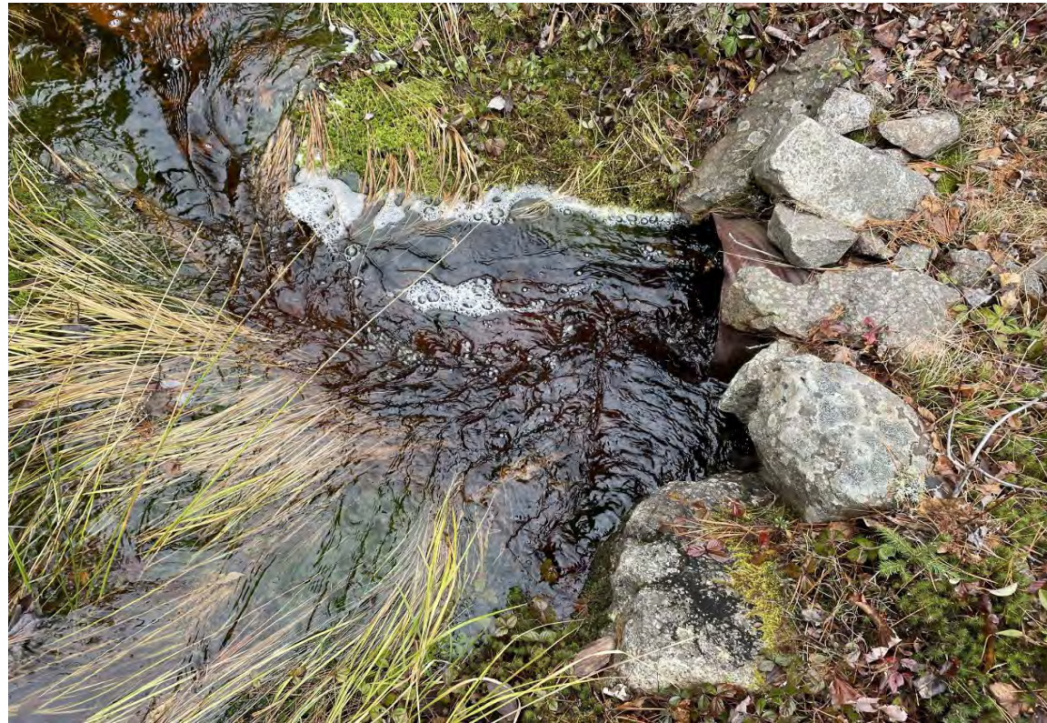
Photo 1: Upstream at Crossing Location with Culvert
