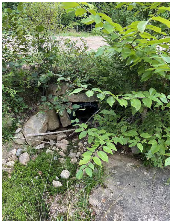
Photo 1: Upstream at crossing, culvert present.
