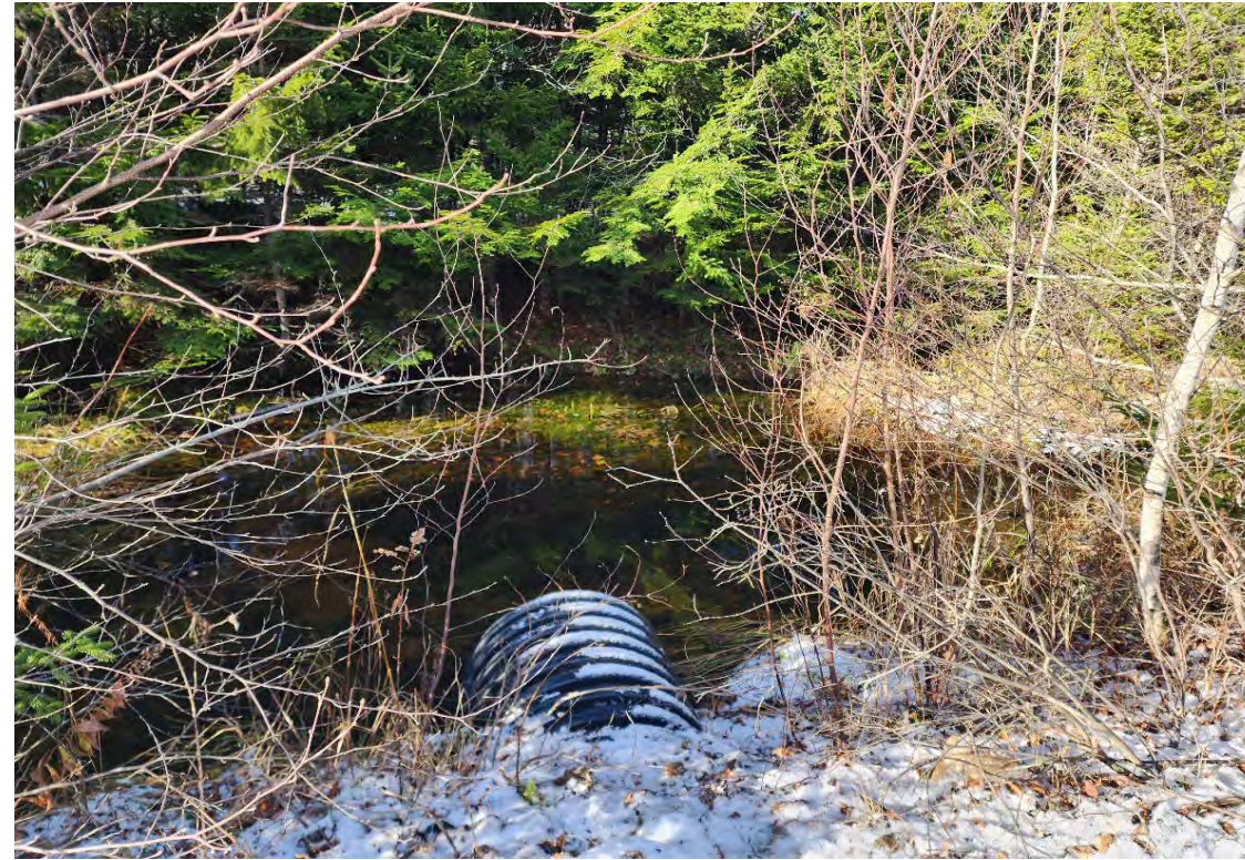
Photo 2: Culvert at crossing Location
