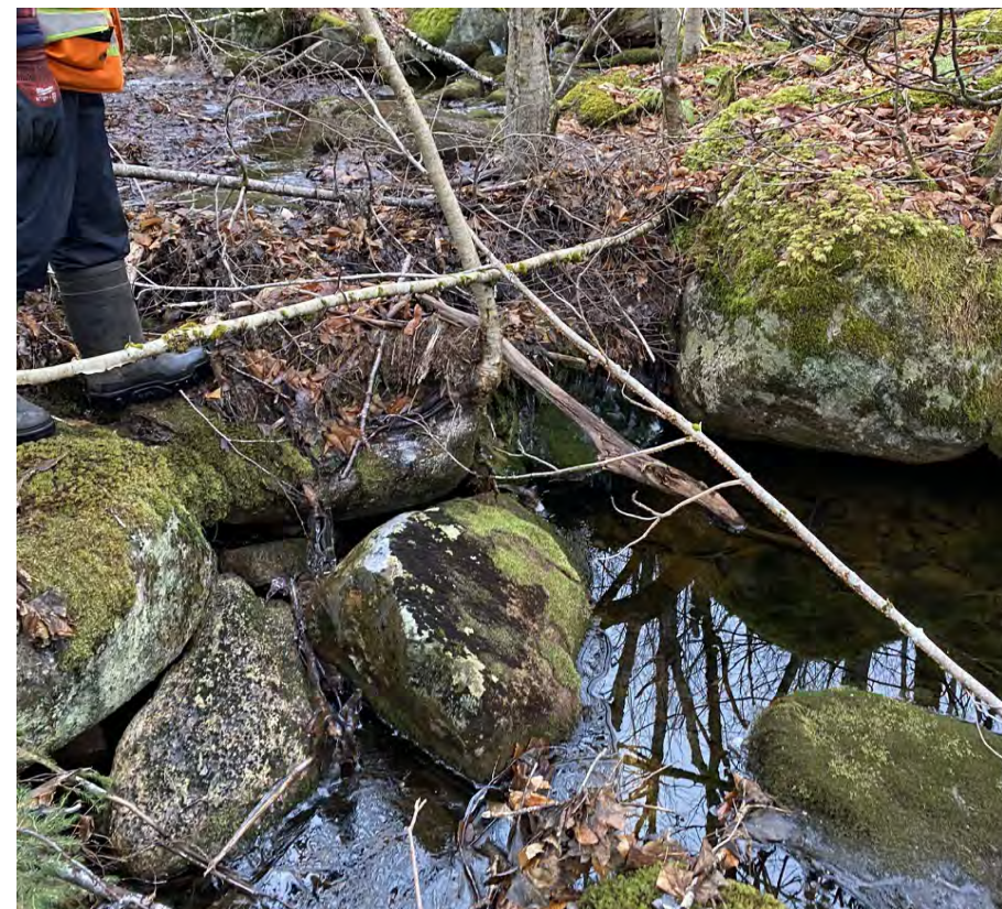
Photo 4: Potential Fish Barrier
