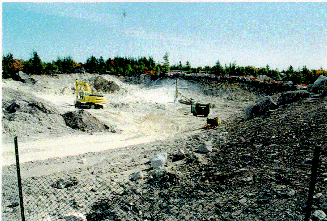
Plate 1: Exploration pit north of Highway 203, October 4, 2000.
