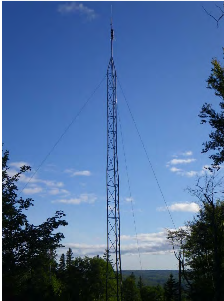
Photo 3.2 Pole erected on site for aerial Anabat system in 2013, showing detail of forest edge.
