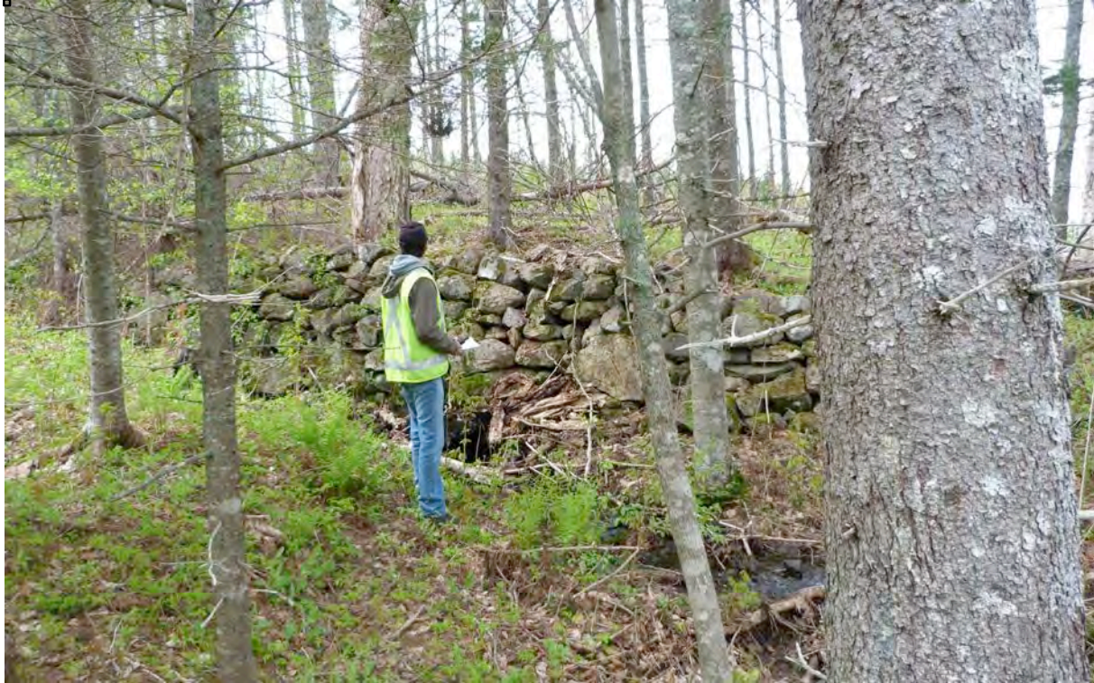
Plate 5: Road retaining wall along east section of old road looking southwest.
