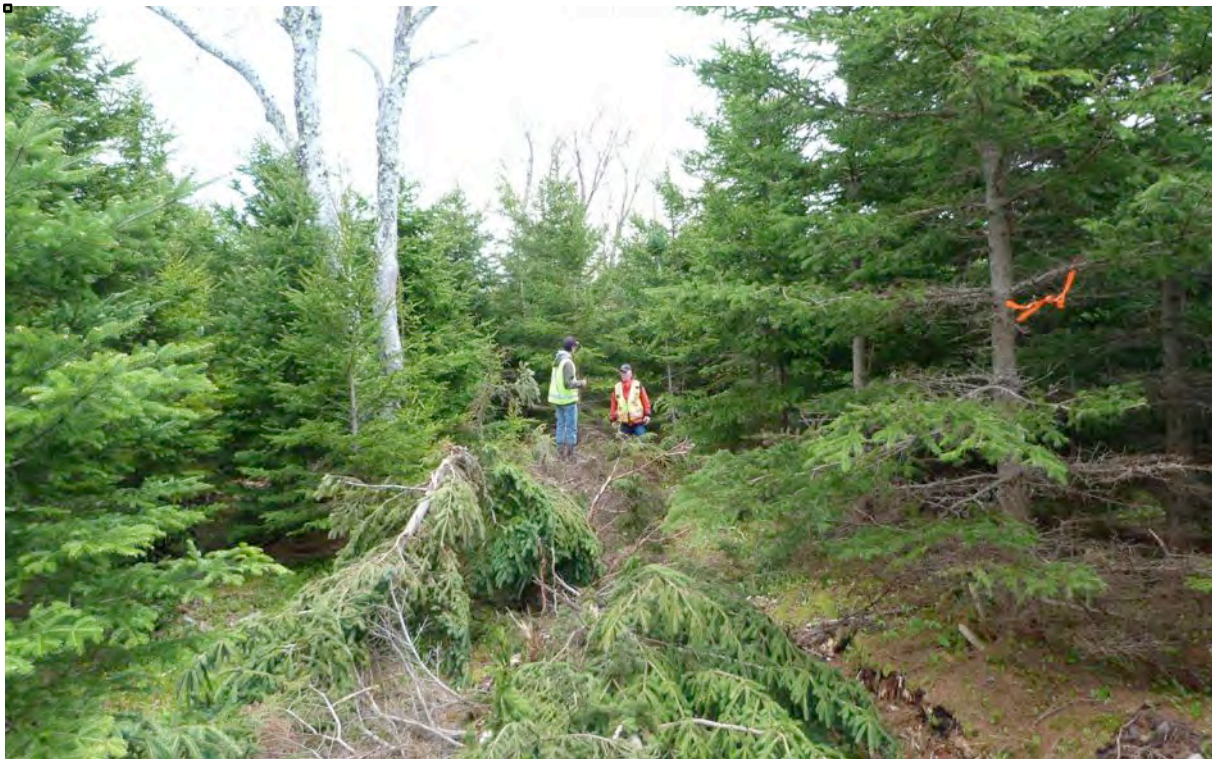
Plate 8: Turbine site two, looking east. Note the survey tape and tree push-out from geological testing.
