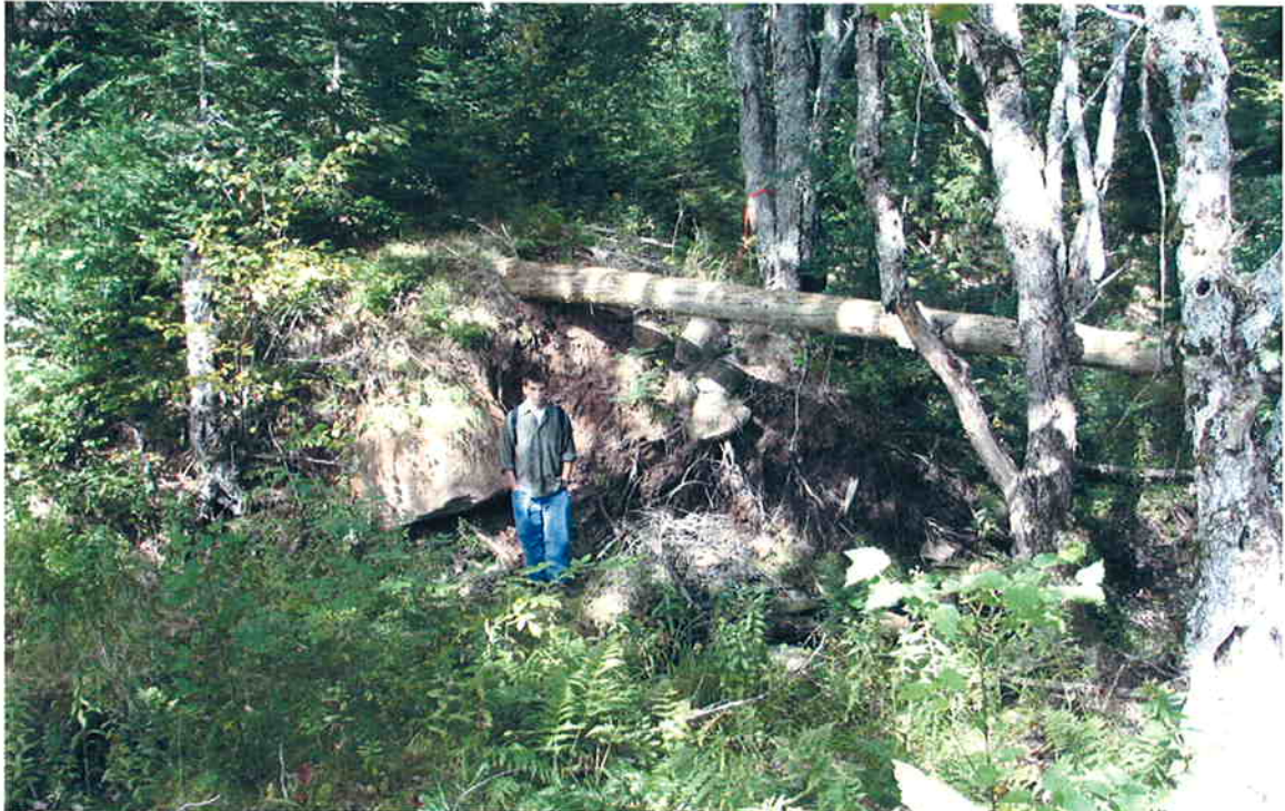
PLATE 9: Breech Dam at the R. Masson Saw Mill Complex.
