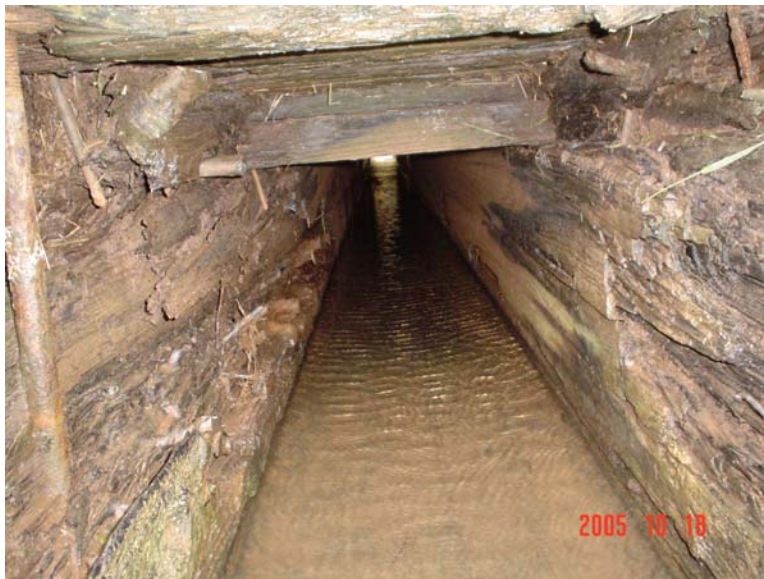
Photo 4: Wooden culvert of tributary, 977m upstream LaPlanche River from bridge
