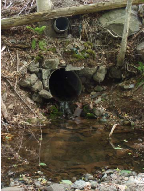
Photo 6: WC-1 - Upstream end of culverts under gravel road (outside project area)
