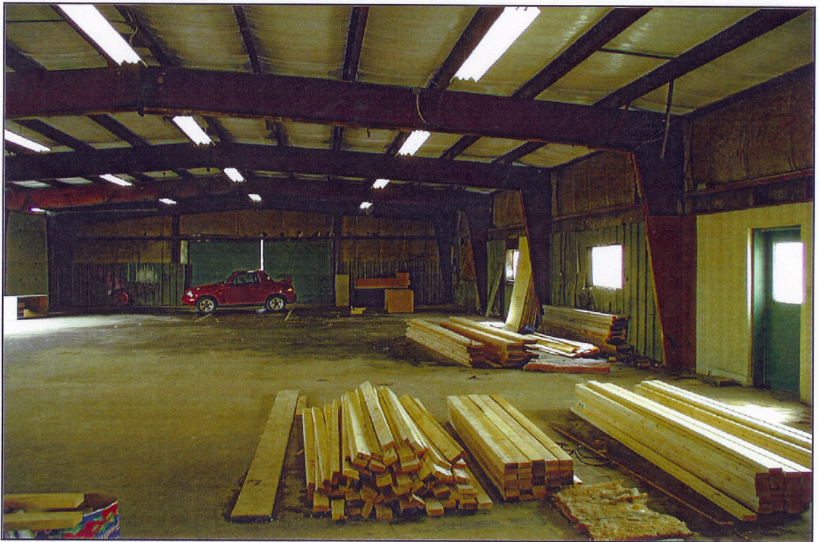
Photo 10 – Inside View of Warehouse
