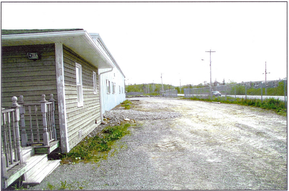
Photo 1 – 533 Rocky Lake Drive – View along Front of Building
