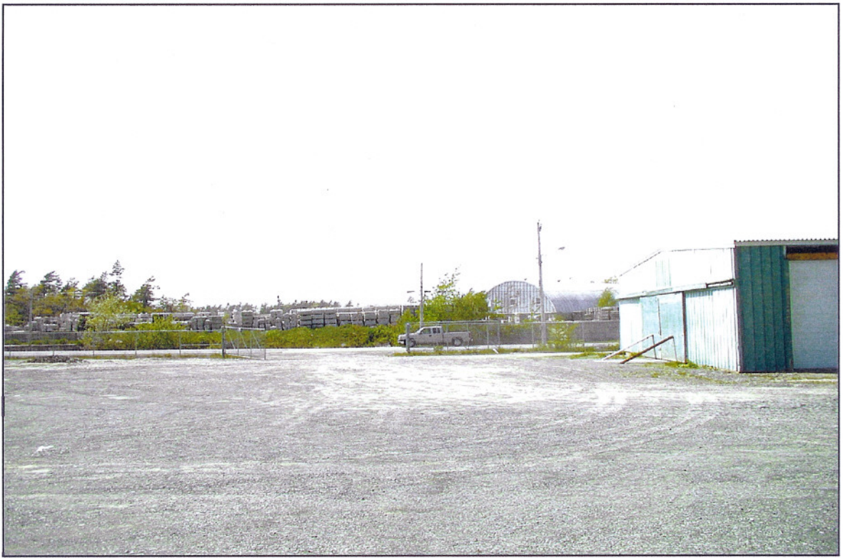
Photo 3 – Side View of Warehouse
