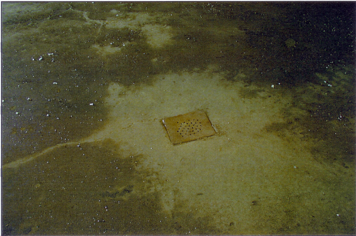
Photo 11 – Floor Drain in Warehouse
