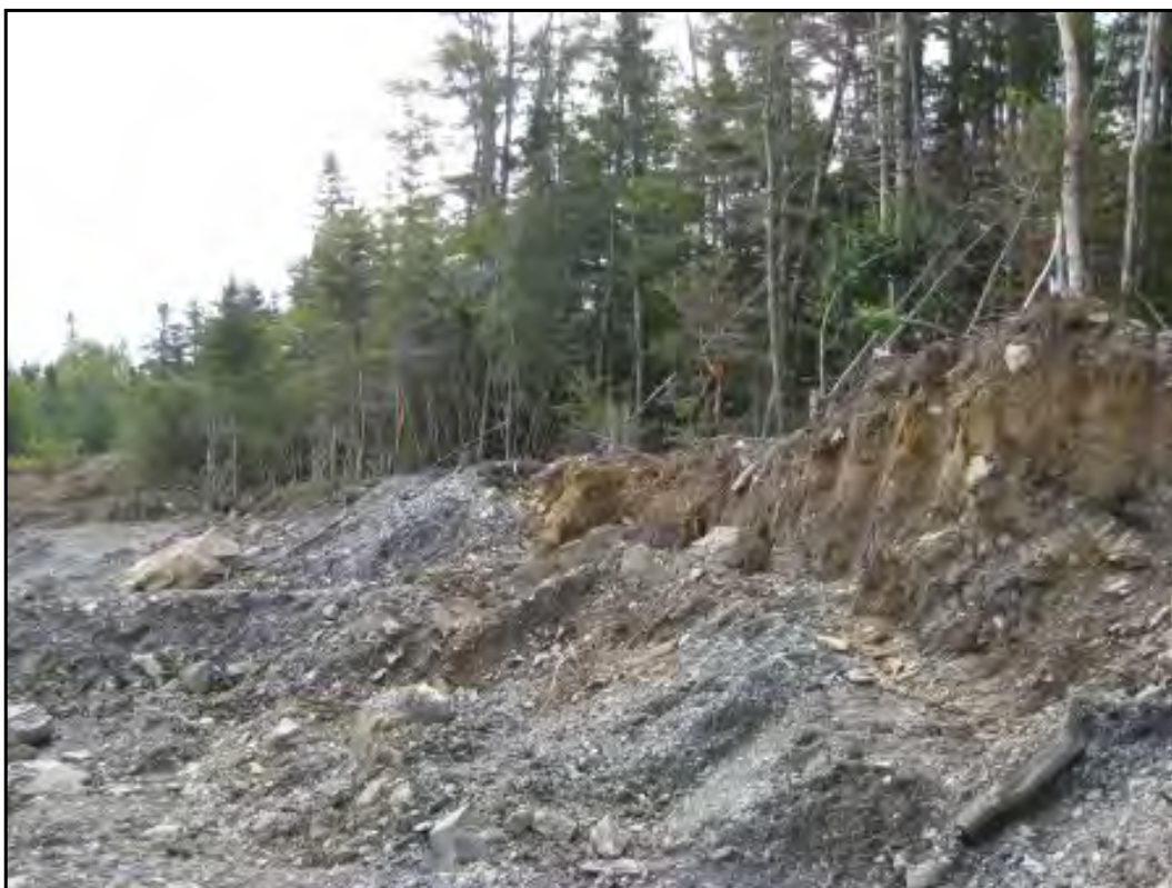
Typical Transition Between Areas That Have had Overburden Removed and Tailings Areas
