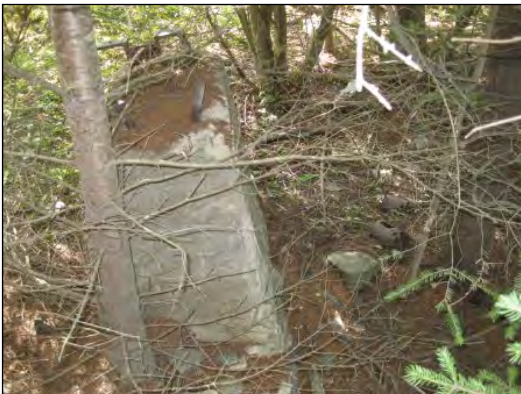
Foundation Remains of the Moose River Gold Mine Stamp Mill (Crusher)
