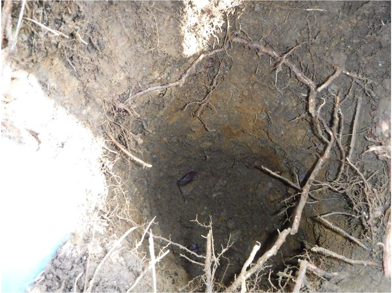
Figure 3 GK17-BH20. Possible tailings were not identified at this location. The following materials were identified: at 0-0.05m BGS a black organic rootmat and at 0.08-0.68m BGS a poorly sorted brown grey silty sand and gravel with cobbles.
