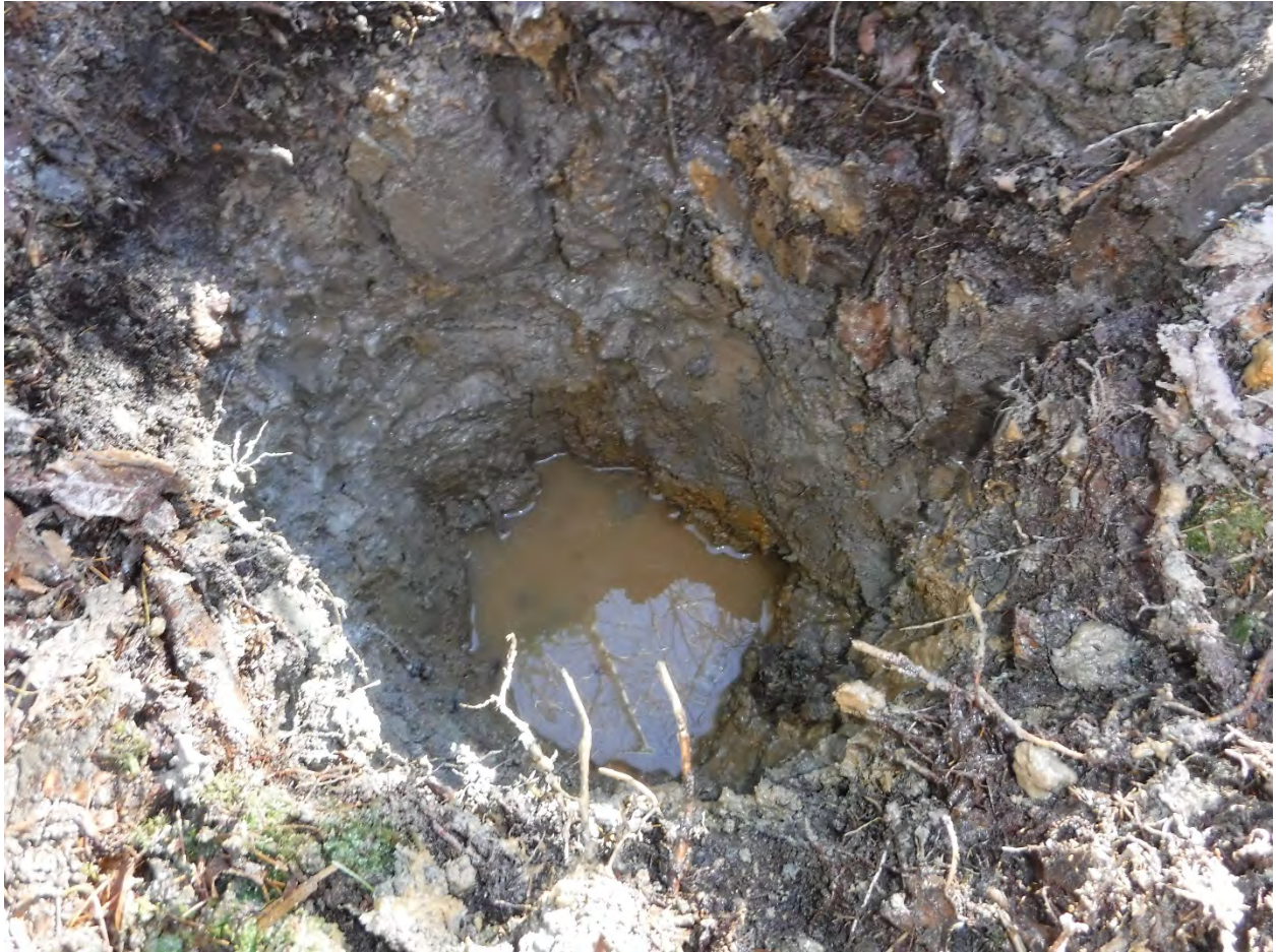
Figure 4 MR17-BH19. Possible tailings were identified in this location. The following materials were identified: at 0-0.08m BGS an organic rootmat, at 0.08-0.30m a well sorted grey silt with interspersed large cobbles (possible tailings) and at 0.30-0.55m a poorly sorted brown silty sand with cobbles.
