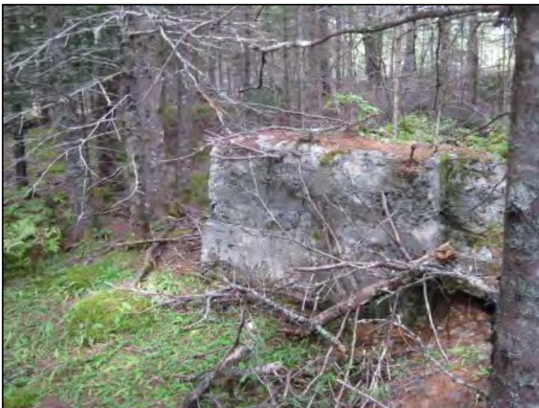
Foundation of the G&K Stamp Mill (Crusher)
