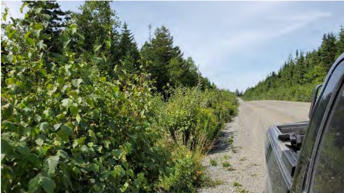
Photo 5: TSP 5 located near the shoulder of Mooseland Road.
