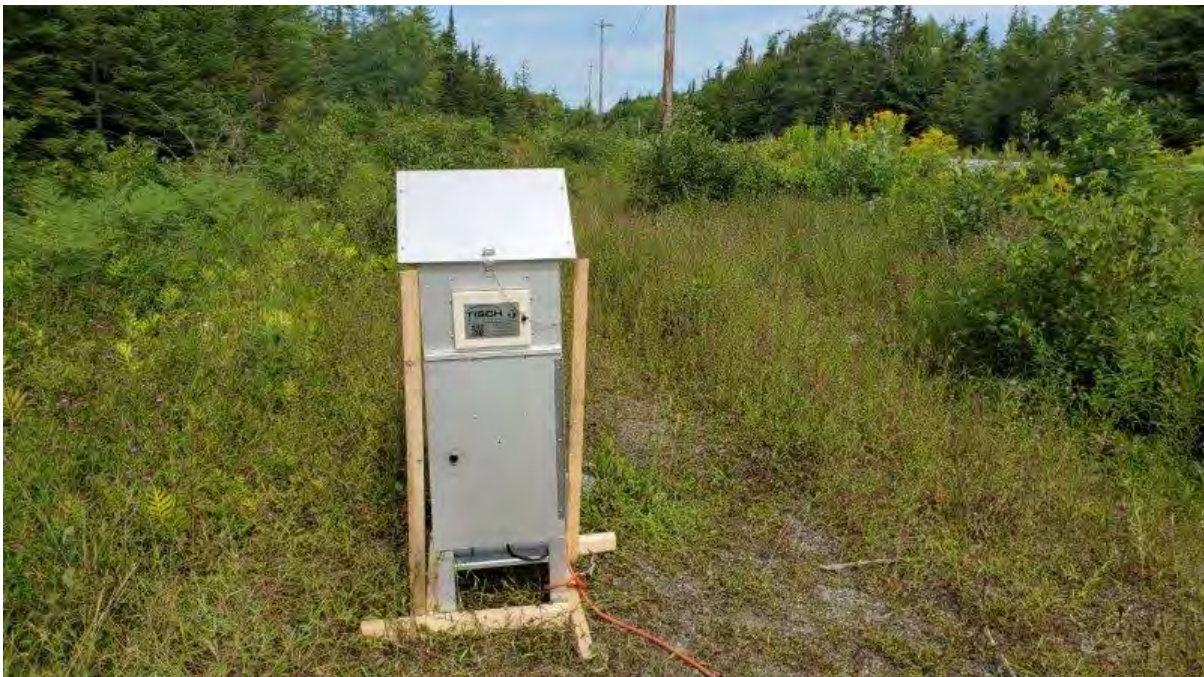
Photo 4: TSP 4 located near the shoulder of Mooseland Road.
