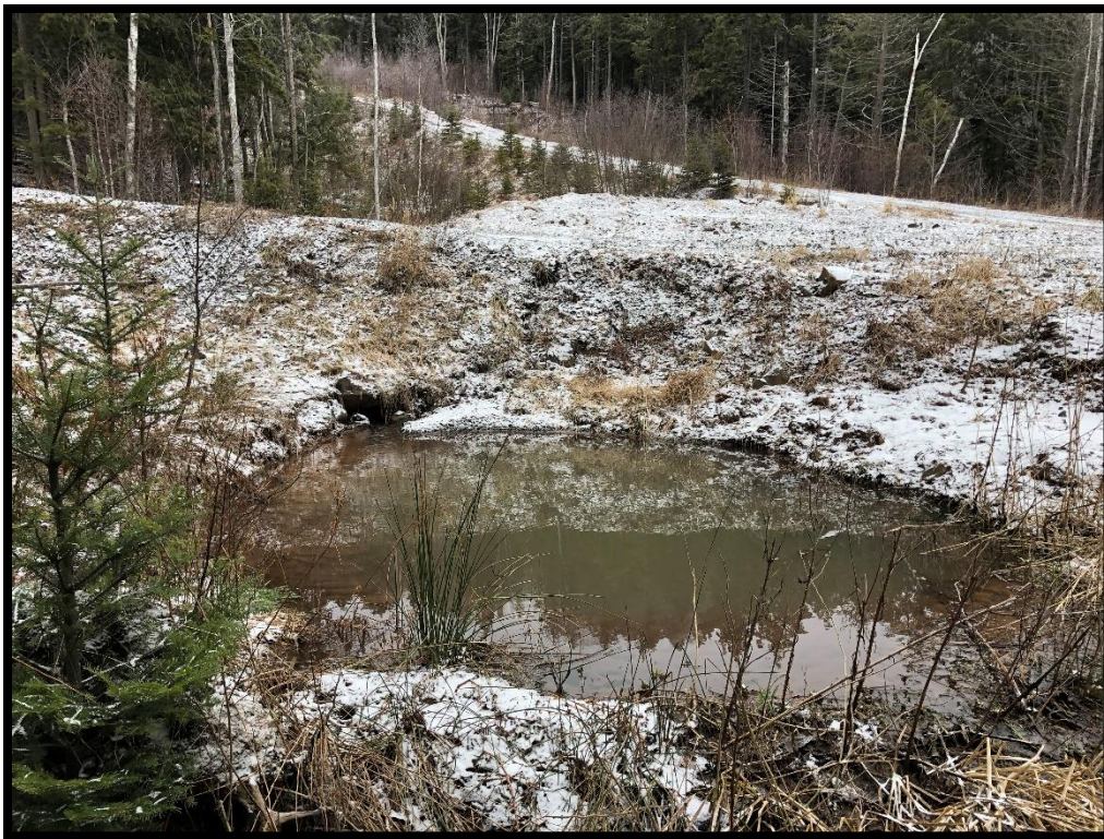
Figure 7: A sediment catch basin collects ditch drainage and any potential sediment along the OHV access road.
