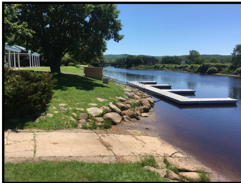
Figure 43: Jubilee Park Boat Launch and Floating Wharf, Bridgetown
