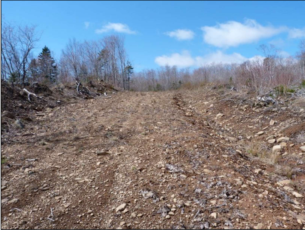
Plate 1: A bulldozed road leading westward in the northwest quadrant.
