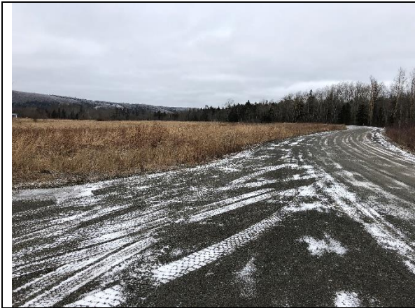
Photo 1: Entrance of access road to Spicer Quarry from Highway 1. The active and proposed quarry are located at the top of the north mountain in the distant portion of the photo. Note stone cover on the access road to limit tracking of dirt onto Highway 1, and old field habitat.
