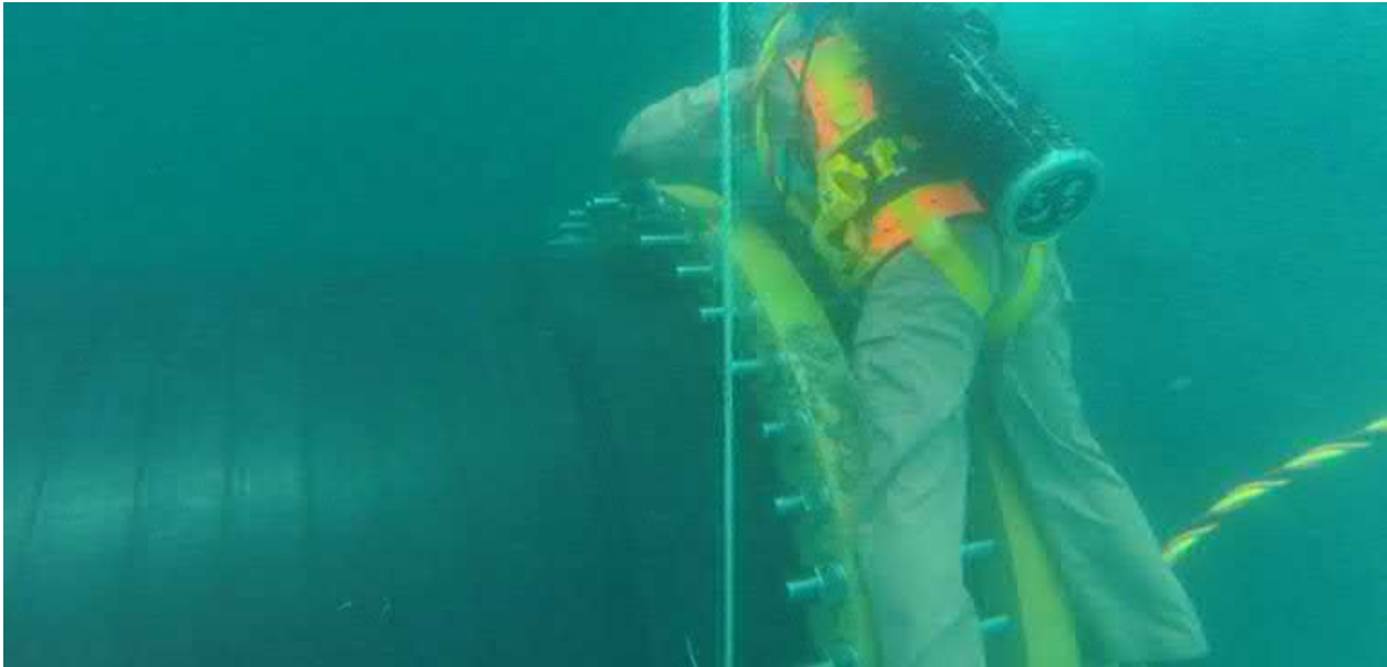
Figure 32. Diver working on HDPE pipeline connection.
