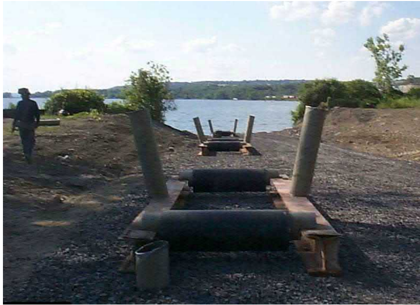
Figure 22. Roller beds used to move fused pipe down to the water.
