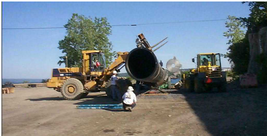
Figure 21. Loading pipe (63") into fusion machine with front end loader.
