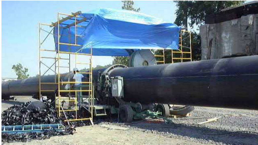
Figure 20. Fusion machine set up to fuse 63" HDPE pipe.
