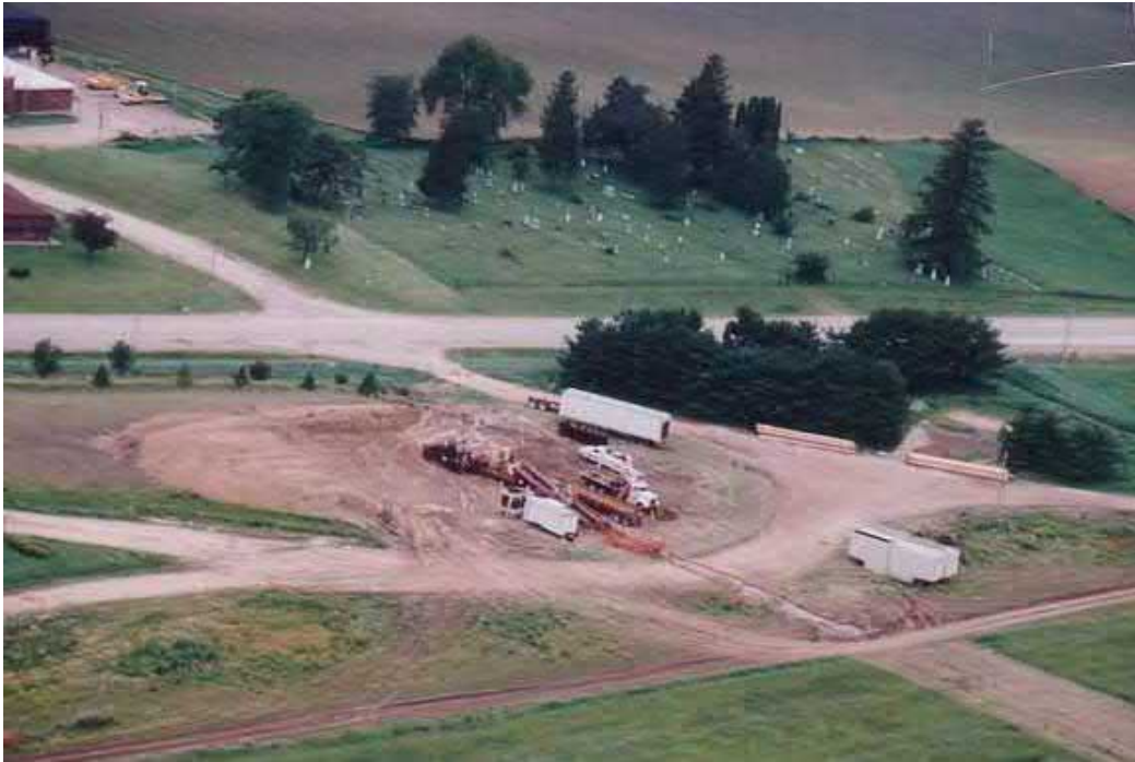
Figure 34. Aerial view of HDD in progress.
