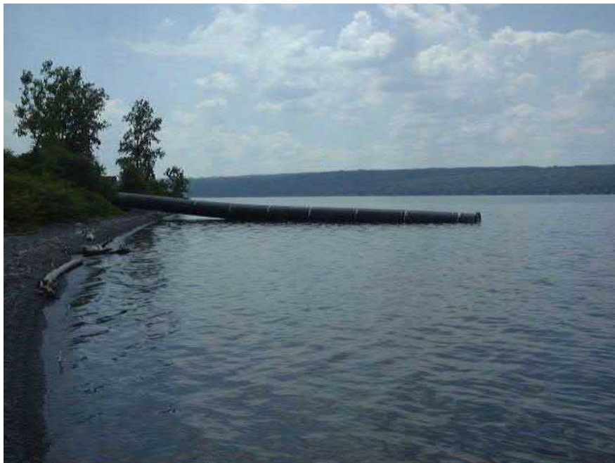
Figure 23. Fused pipe (63") entering the water.
