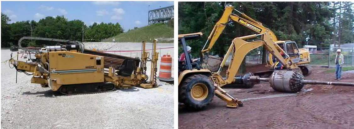
Figure 33. HDD drill rig (left) and reaming head (right).
