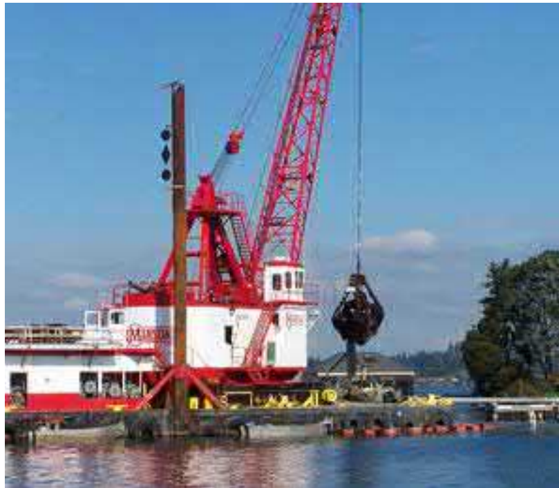
Figure 11. Example of typical clam-shell excavator, taken from Manson Construction website, http://www.mansonconstruction.com/andrew/..
