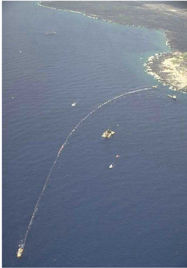
Figure 30. Deep water pipe deployment – maneuvering to counter cross-currents.
