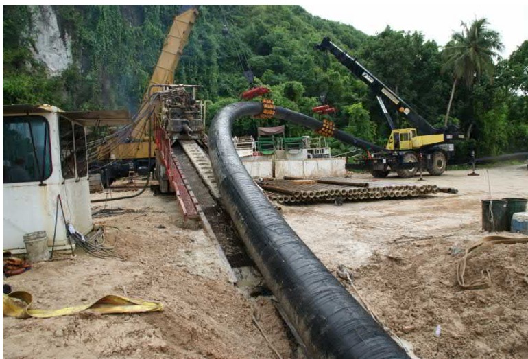
Figure 35. Example of HDPE pipe being placed via Horizontal Directional Drilling.
