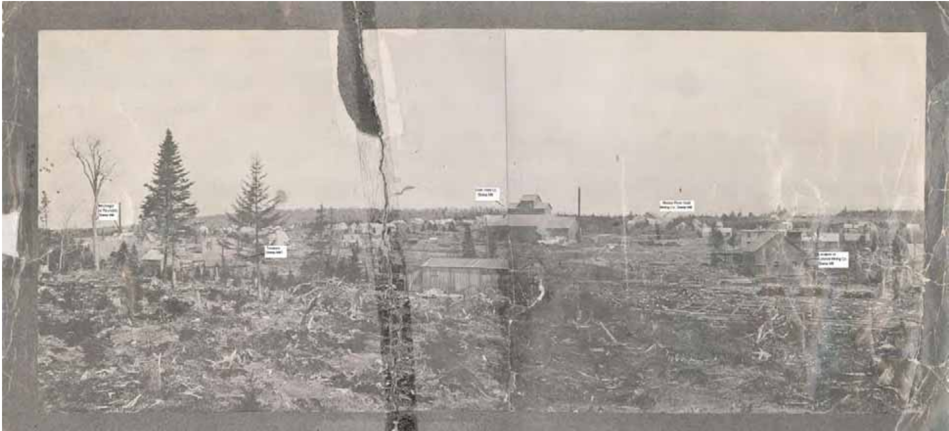
Figure 2 – Moose River Gold Mines (looking east from the west bank of the Moose River)
