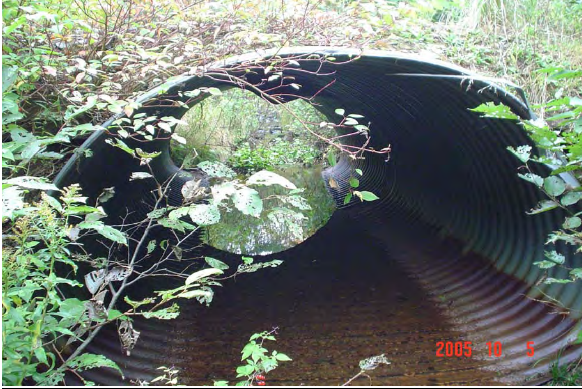
Photo 1: (Stream A) Closed bottom metal culvert
