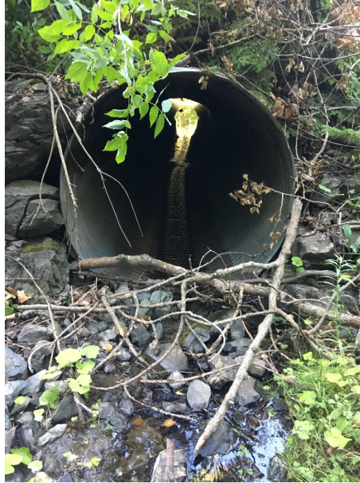
Waypoint 1: Culvert beneath Quarry Access Road, looking downstream from culvert inflow.
