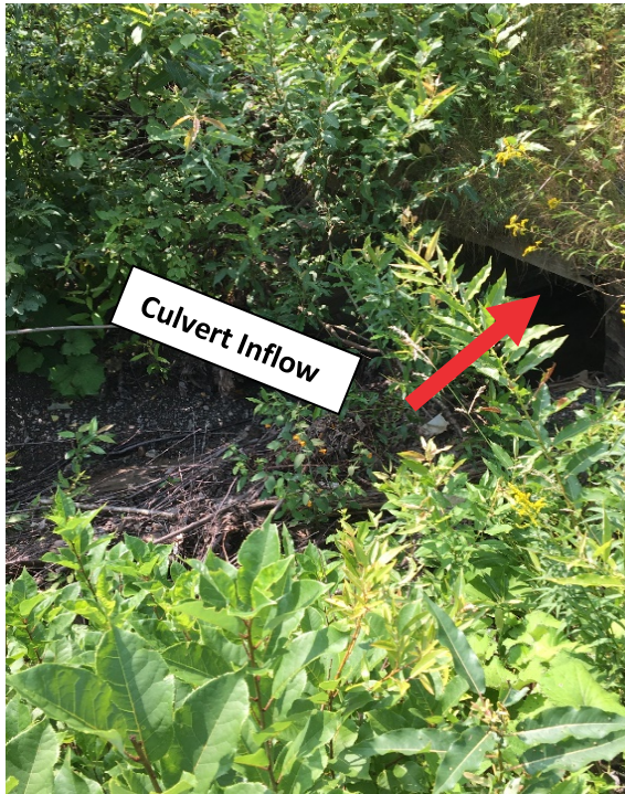
Waypoint 25: Debris pile at inflow of culvert beneath McLellans Mountain Glencoe Road. Debris pile assessed as a barrier to fish passage.
