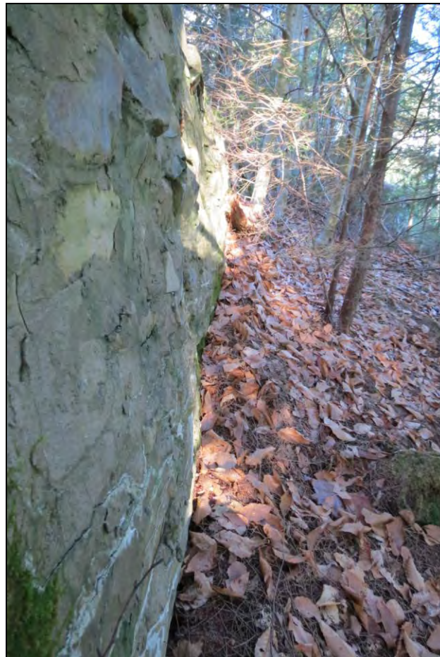
PLATE 14: Retaining wall located on Potential Impact Area C-2. Facing north. December 5, 2014.
