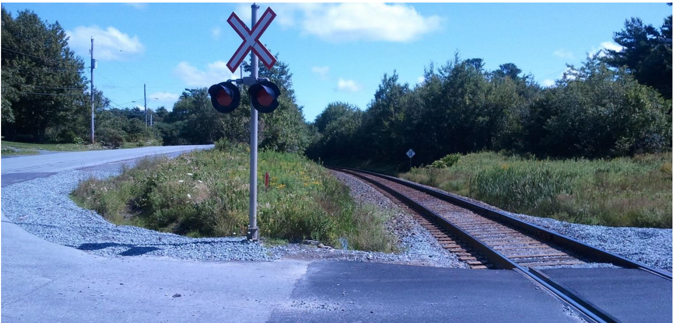
Figure 5: Sunnylea Rd Looking North along CN Tracks
