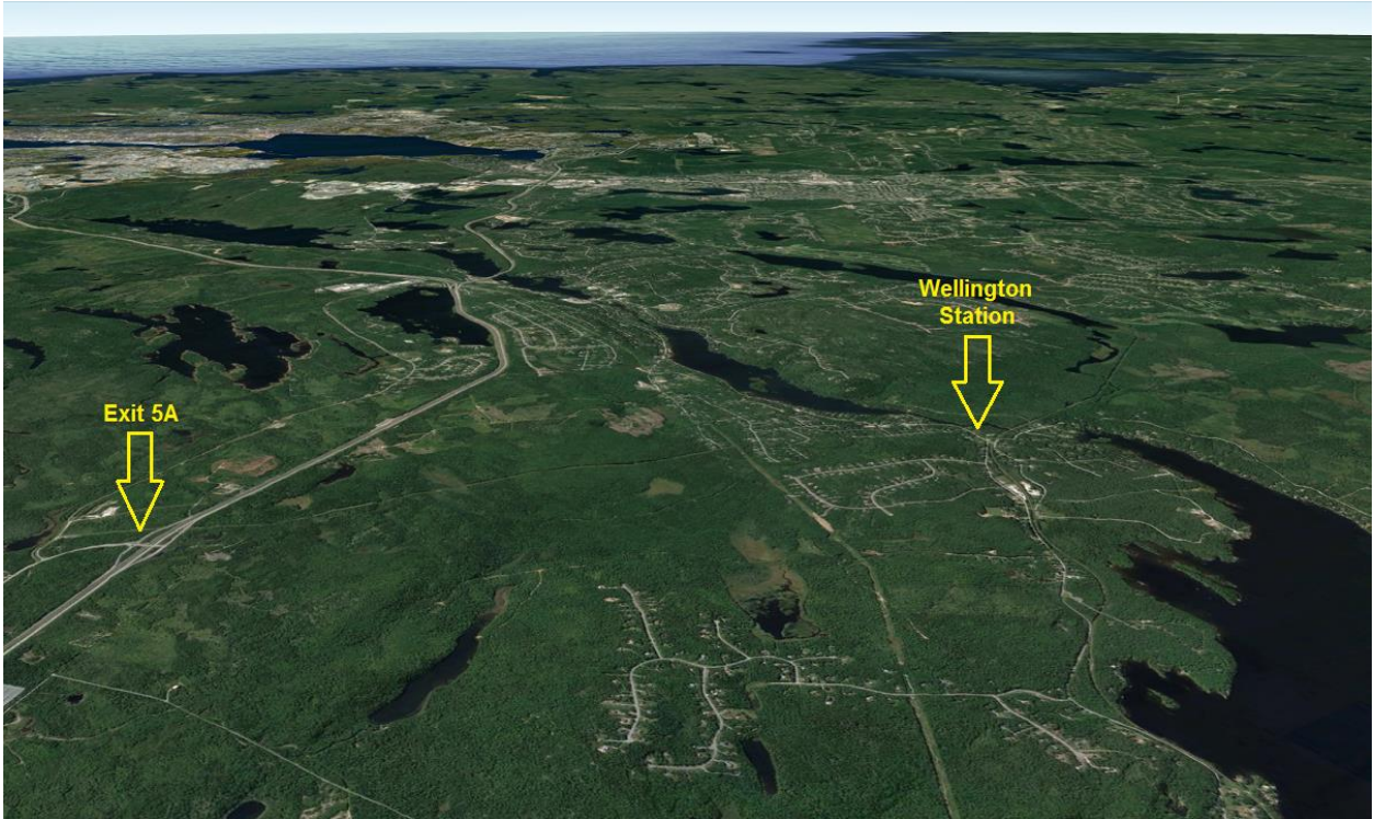
Figure 3. Project Site Looking South
