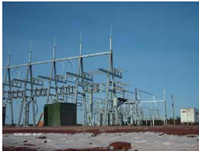
Photo 11. Substation under construction with 4 collection system circuits.
