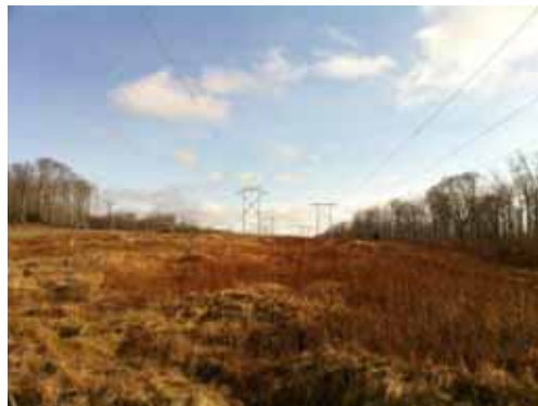
Photo 2. Existing NSPI transmission line through south end of Project lands
