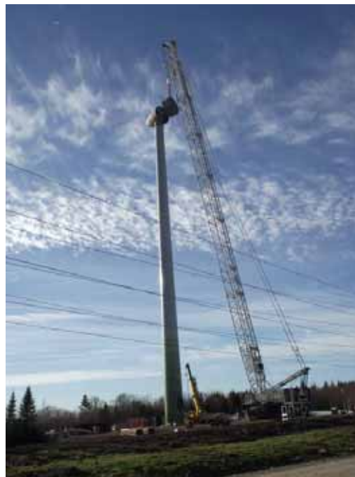
Photo 9. Nacelle Installation
