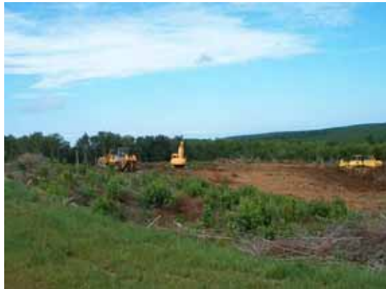
Photo 5. Typical clearing operations of a turbine site following timber removal
