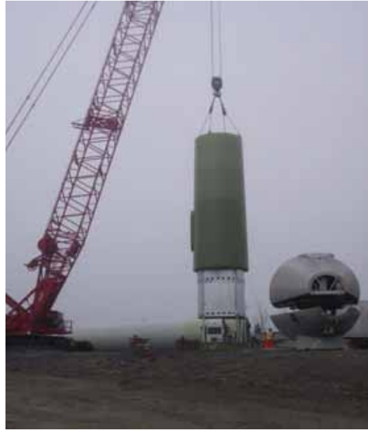
Photo 8. Tower section installation
