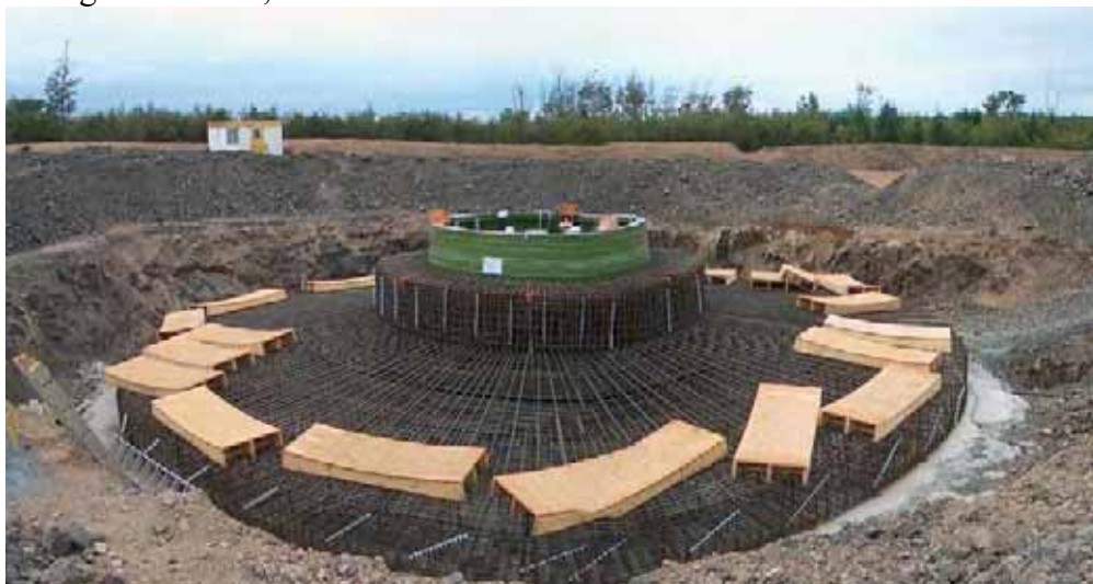
Photo 6. Typical turbine re-bar installation for the spread foot foundation.
