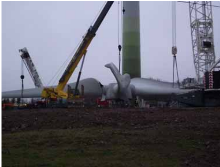
Photo 10. Hub and Blade Lift.
