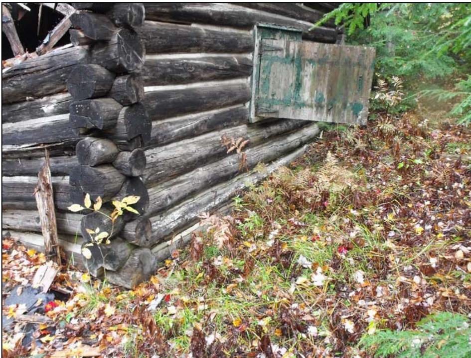
Plate 14: An abandoned cabin near the study area, resting on wooden sills on the ground likely in the same style of many pioneer structures. Looking north.
