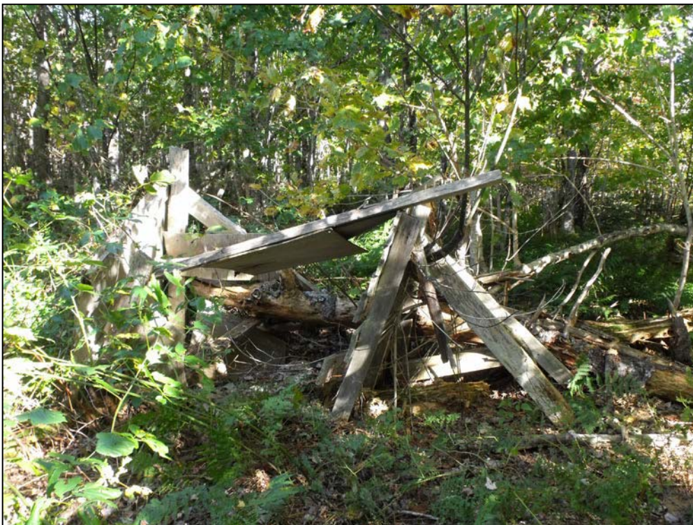
Plate 12: A collapsed hunting blind near the access road to turbine candidate 62. Looking east.
