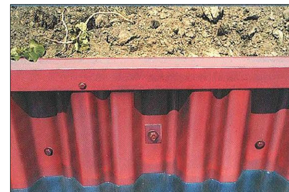
PHOTO EXAMPLE OF SHEET PILING
