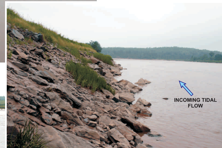
3. Close-up of riprap on the dike.
