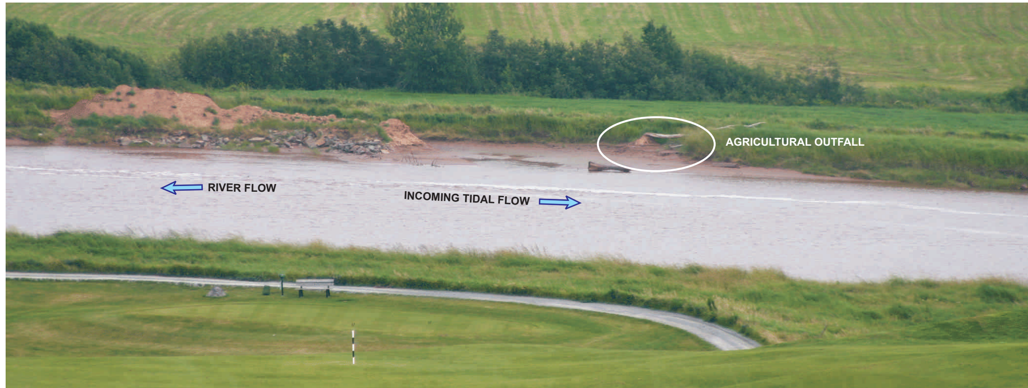
1. Embayment in bank (reportedly used as an outfall area to the river).
