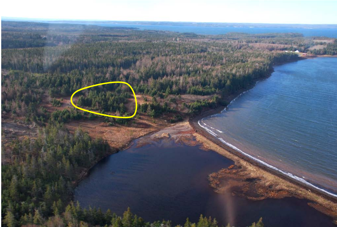
Plate 7-1: Oblique aerial view of the Janvrin Island site looking southeast (2009) – courtesy of NSE.
