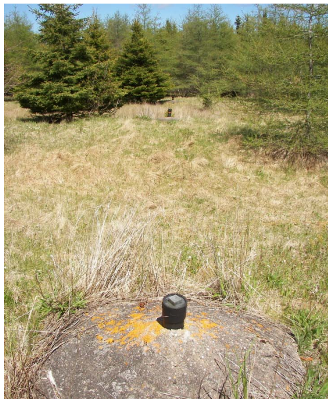
Plate 5-3: Tree growth over the cover caps and around the in-trench monitoring wells for Trenches 2 (foreground) and 3 (center background) on 26 May 2010.
