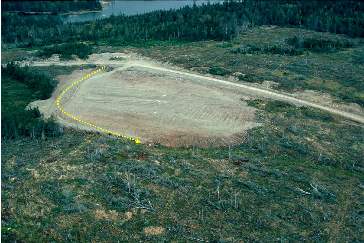
Plate 5-5: An oblique aerial view of the site after capping looking toward the northeast. Note the French drain and swale diverting shallow groundwaters around the site.
