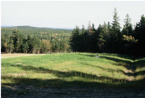
Plate 5-6: An oblique aerial view of the site after capping, looking toward the northeast. Note the French drain and swale diverting shallow groundwaters around site.
