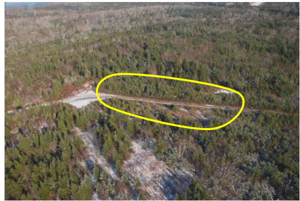
Plate 5-2: Oblique aerial view of the Hadleyville site during this assignment (2009) looking north.
