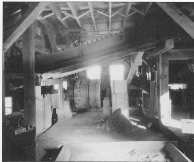
Interior of the milling house of the Lacey gold mine at Gold River gold district in Lunenburg County, Nova Scotia, 1934. The conveyor (top) brings rock to the surface where it is crushed and then treated in the amalgamation tray with mercury to separate the gold (foreground).
