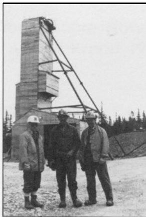
Shaft (background) which provides vertical access to the Forest Hill gold deposit operated by Seabright Resources Incorporated. Underground development presently goes to the 200 m level.
