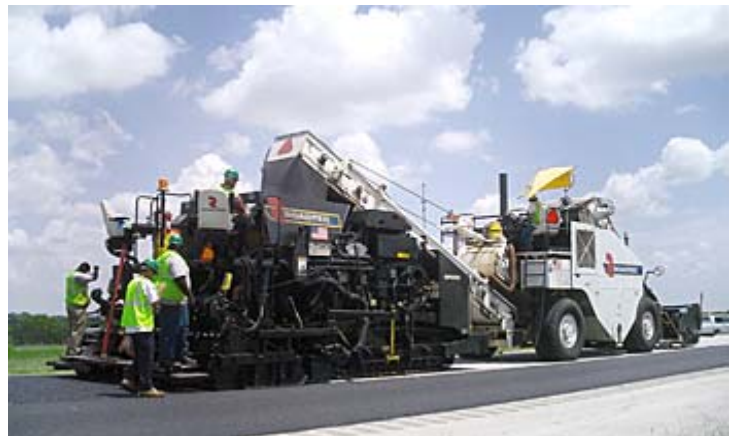
Typical shuttle buggy at work; note position of operator
