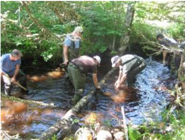
Volunteers with the Port Morien Wildlife Association place digger log in MacVicar's Brook
