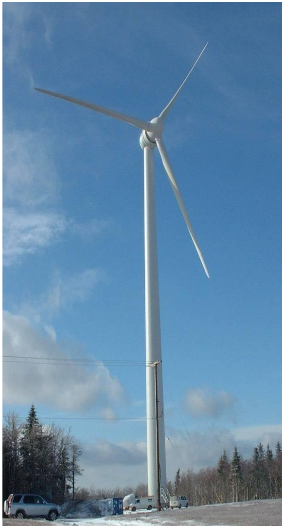
Vensys 1.2MW installed by Eon WindElectric
