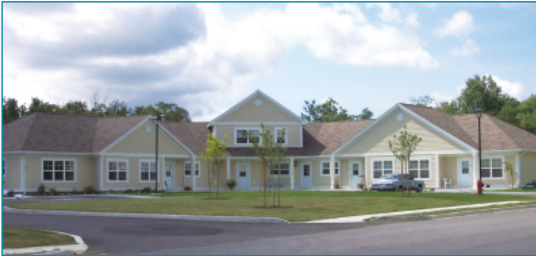
◀ A 15-unit townhouse complex was constructed in Middleton under the New Rental Housing Initiative
