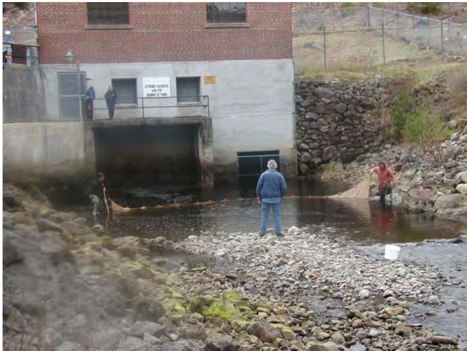
Figure 3.7 Powerhouse seine and ichthyoplankton sample site
