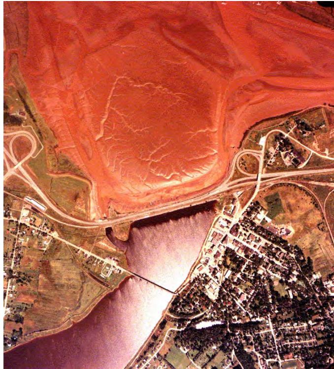
Figure 1.1 Aerial view of the Windsor Causeway, 1981.
