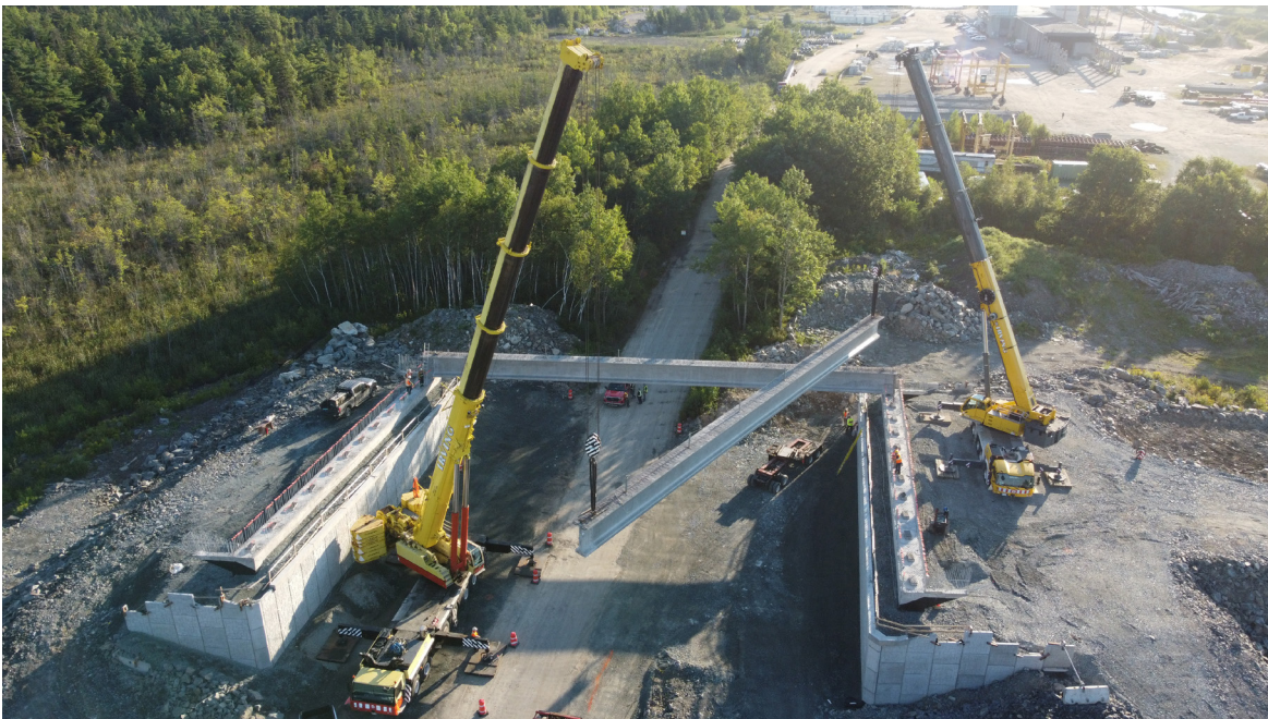
Hwy 107 – Drysdale Ave Overpass
