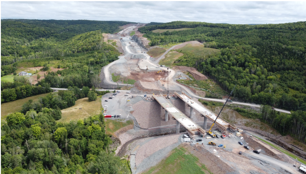
Hwy 104 Middle Brook Bridges
