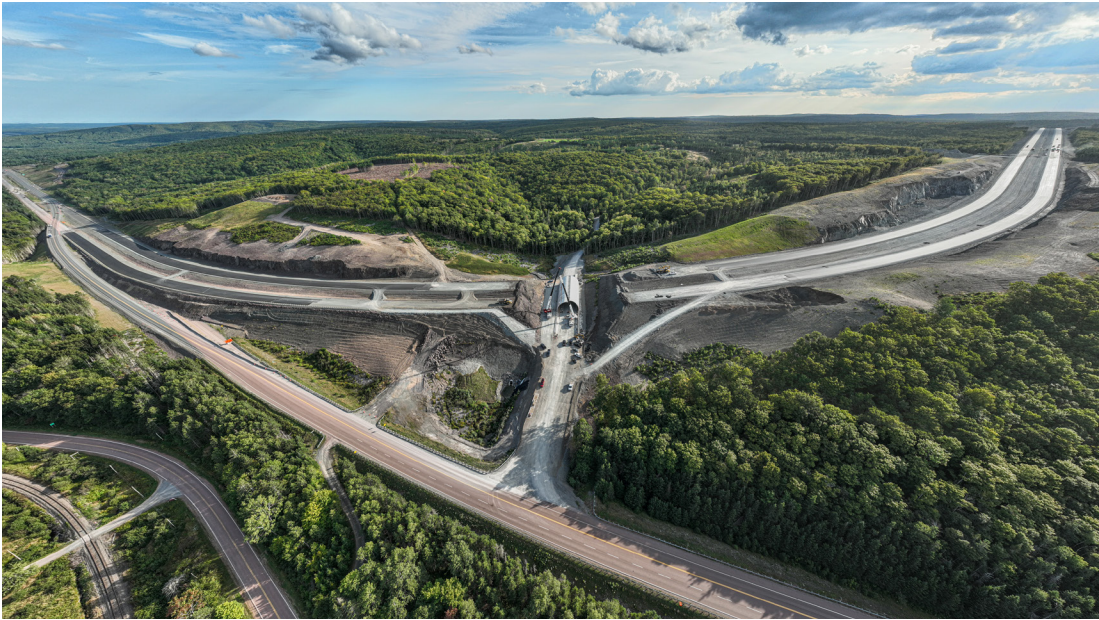
Hwy 104 Pushie Road Arch and Weaver Mtn bypass.
