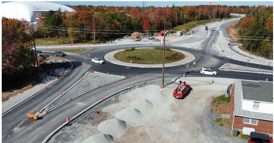
Construction of the Trunk 2 Roundabout in Lantz – October 2021
